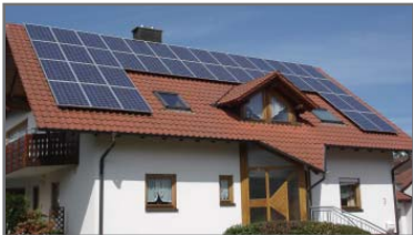
Off-grid home solar system
